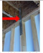
This metal strap goes thru the floor and is attached to the upstairs framework. Nothing wrong, but the inspector has never seen a house that had a metal strap going from the first floor to the second through the floor.
