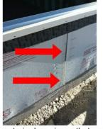
The exterior has pieces that are not sealed. Daylight comes through the gaps. The house should be sealed / wrapped to prevent the entry of insests or moisture.
