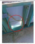
The exterior has pieces that are not sealed. Daylight comes through the gaps. The house should be sealed / wrapped to prevent the entry of insests or moisture. Multiple places around the house did not seal, theymoved and allowed daylight through them. The house should be sealed. ALL exterior openings, not in the plans, should be corrected.
