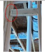
The boards should fill the voids they are meant to be attached between. This board has four nails in it, and it was cut too short. It should have been cut to the correct length, before it was attached. There are a lot of nails that missed their target.
