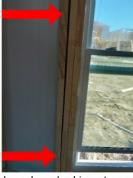
The board marked is not an equal distance from the board next to it. They touch at the bottom, but are seperated at the top. It is beleived they should be touching. It needs to be corrected or explained.
