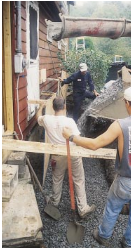
Figure 3. OSB backed with gravel provided a movable form for the stiff concrete mix (left). As the form filled with concrete, additional gravel was dumped against the panels (middle). The OSB was pulled up in one-foot lifts as the pour progressed (right).
