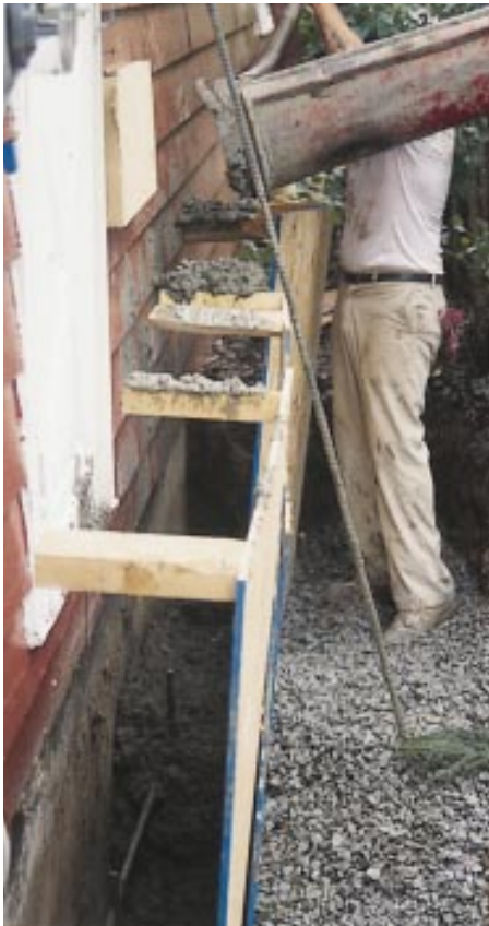
Figure 3. OSB backed with gravel provided a movable form for the stiff concrete mix (left). As the form filled with concrete, additional gravel was dumped against the panels (middle). The OSB was pulled up in one-foot lifts as the pour progressed (right).
