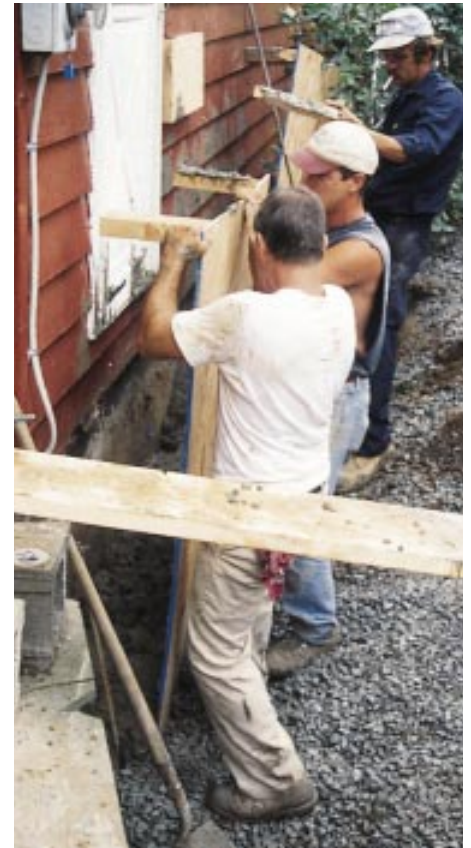
Figure 3. OSB backed with gravel provided a movable form for the stiff concrete mix (left). As the form filled with concrete, additional gravel was dumped against the panels (middle). The OSB was pulled up in one-foot lifts as the pour progressed (right).
