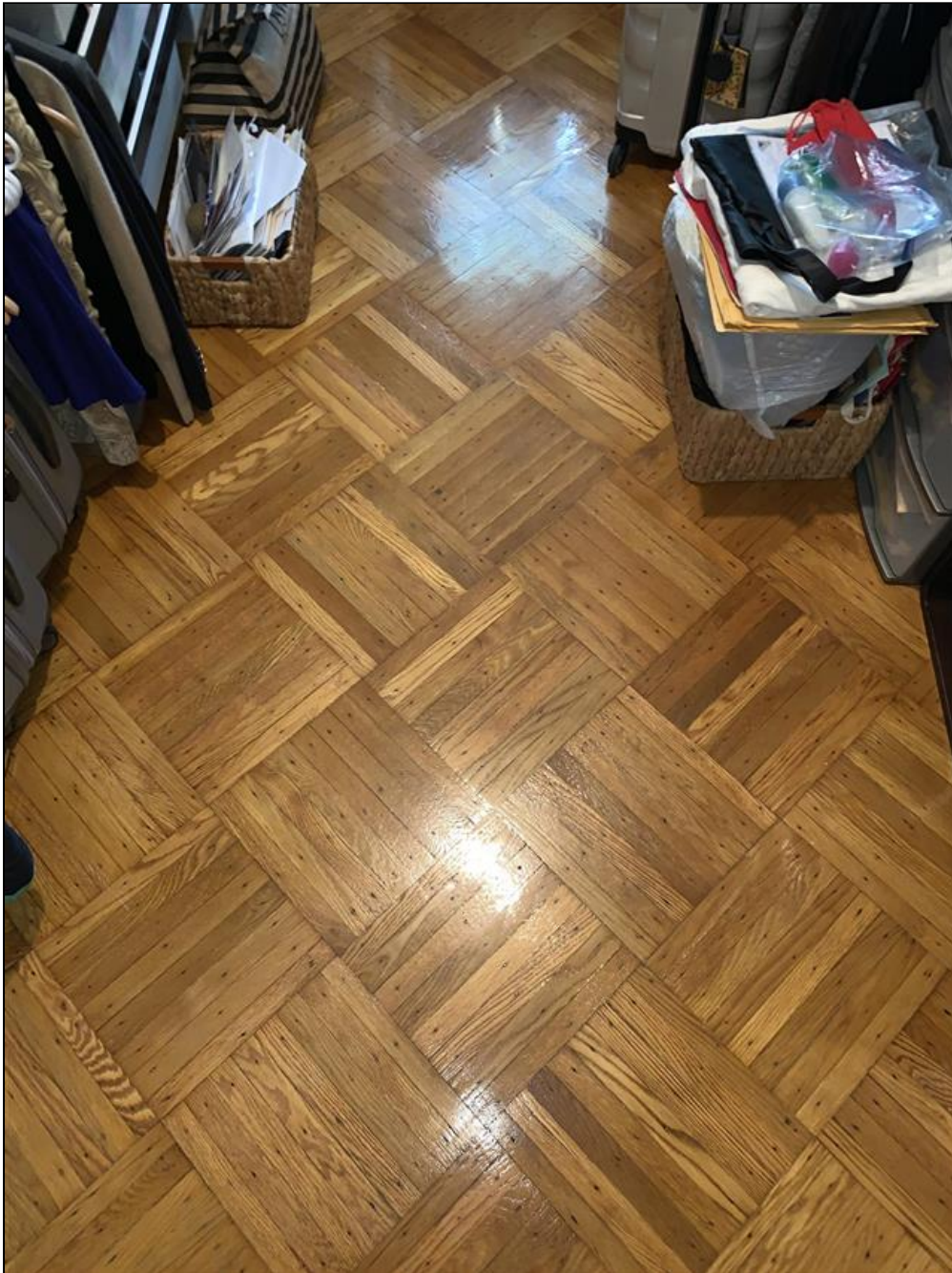
4.2 Item 9(Picture) Third Floor: Example photo of wood flooring.
