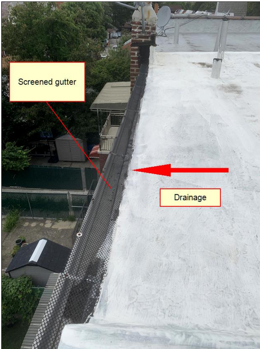
1.3 Item 1(Picture) Photo showing direction of drainage into screened gutter at back of home.
