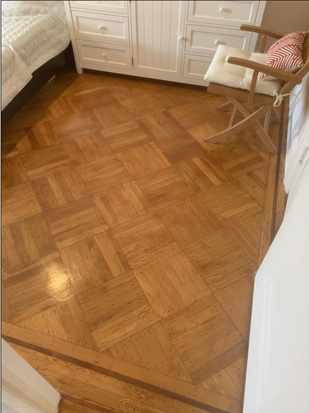
4.2 Item 10(Picture) Third Floor: Example photo of wood flooring.
