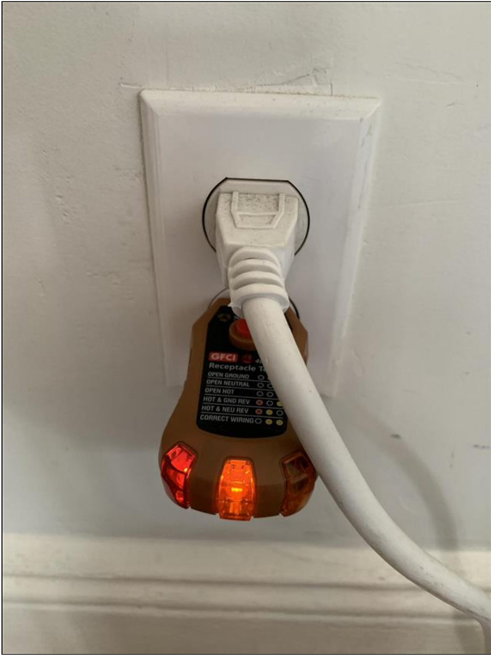
7.3 Item 9(Picture) Hot & neutral wires reversed.
