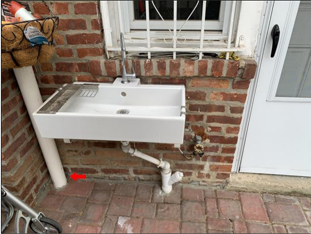
1.3 Item 2(Picture) Downspout from back of roof.
