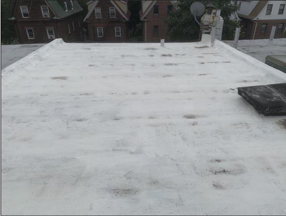
1.0 Item 2(Picture) Roof (facing toward rear of home).
