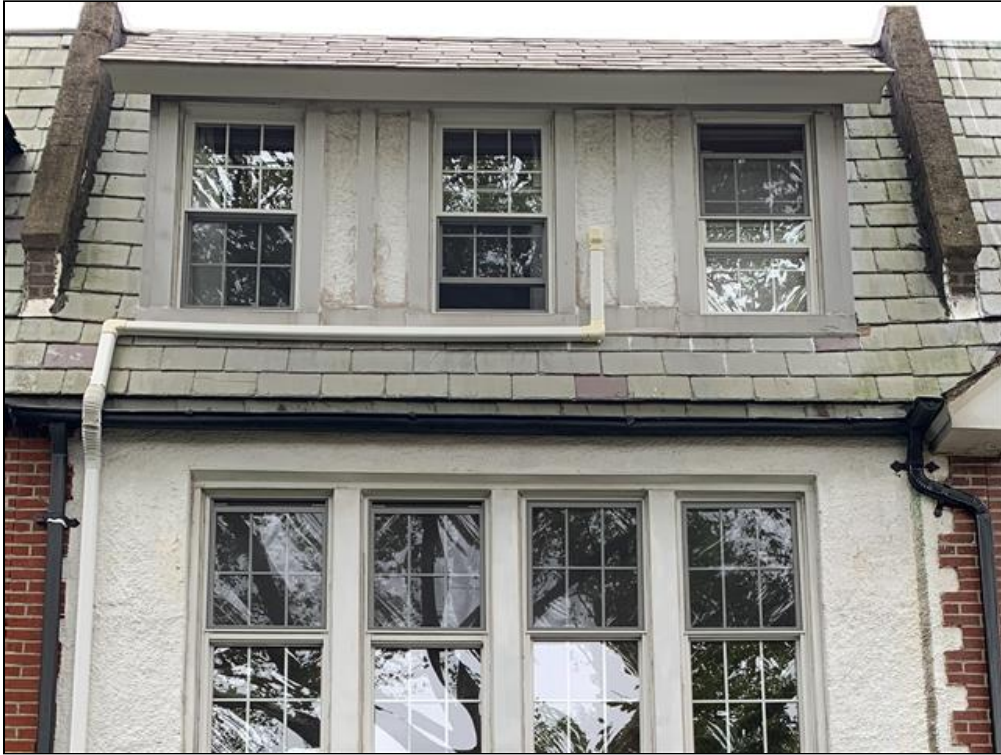
1.0 Item 5(Picture) Slate roof surfaces at front of home.
