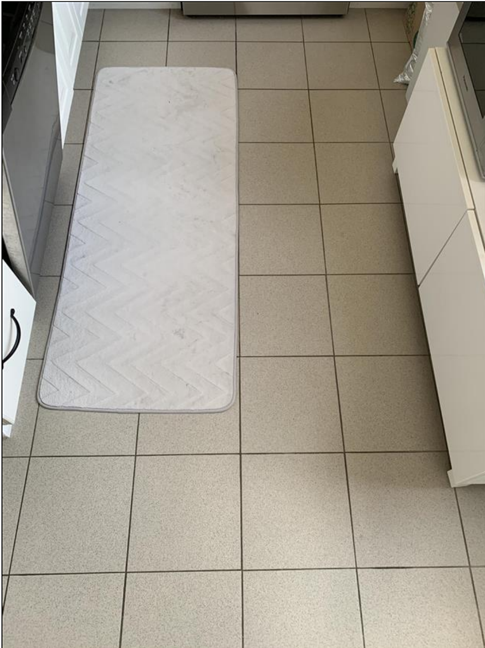
4.2 Item 4(Picture) Second Floor Kitchen: Tiled Floor.
