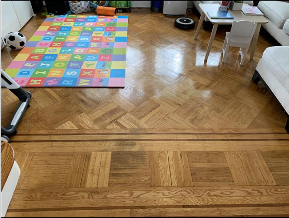
4.2 Item 7(Picture) Second Floor: Example photo of wood flooring.
