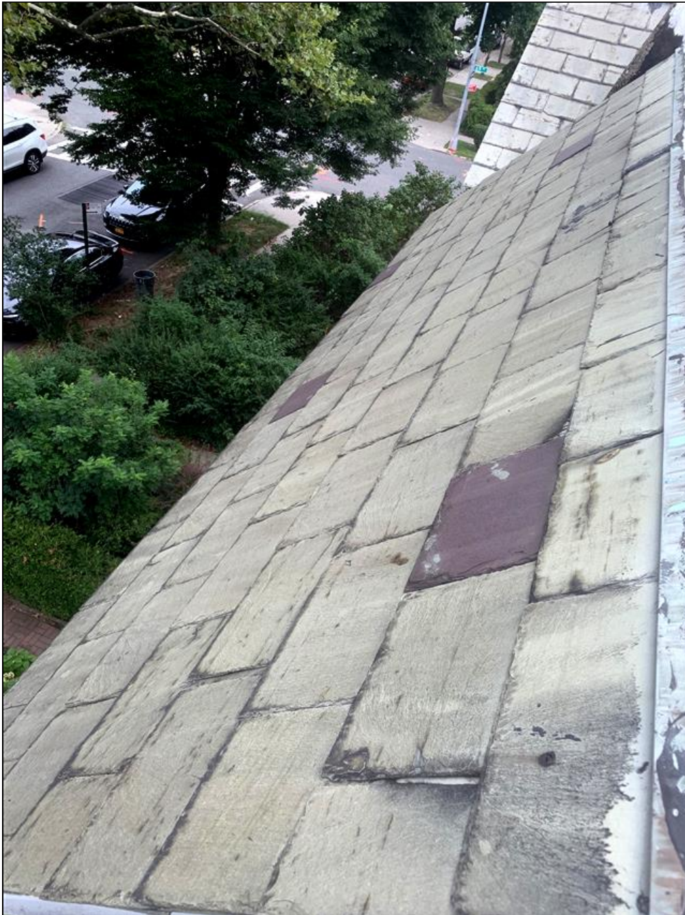
1.0 Item 6(Picture) Slate roof above front third floor windows.
