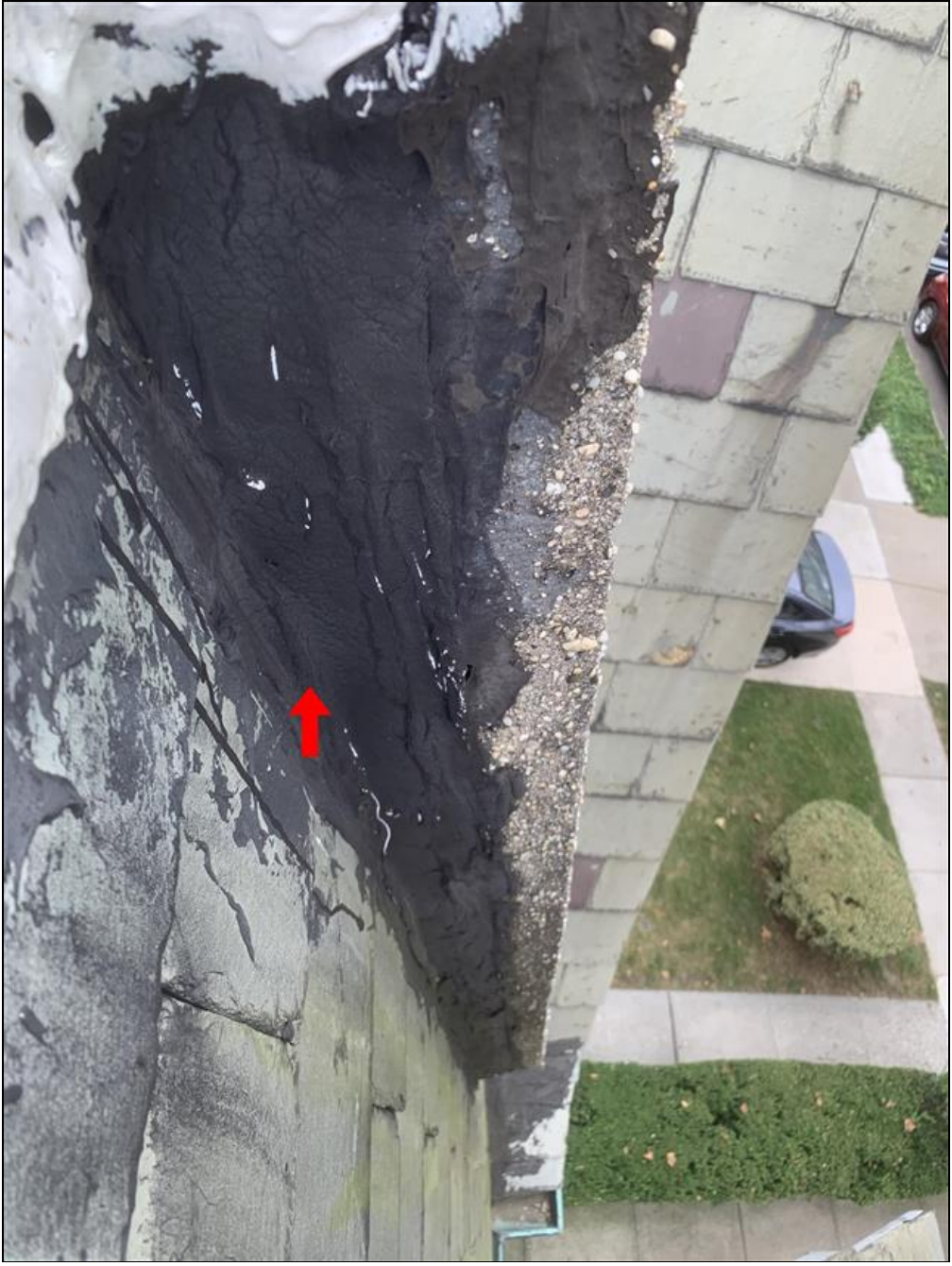
1.1 Item 3(Picture) Flashing cement used here appears to be holding its seal but will eventually need maintenance.
