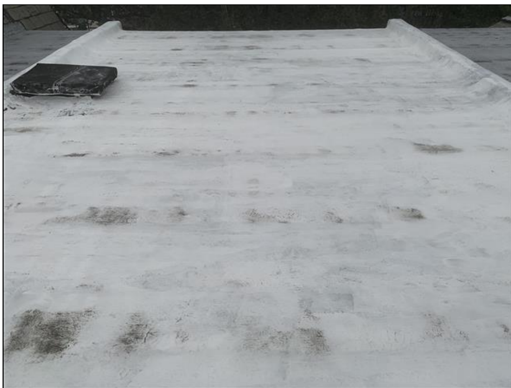
1.0 Item 1(Picture) Roof (facing toward street).
