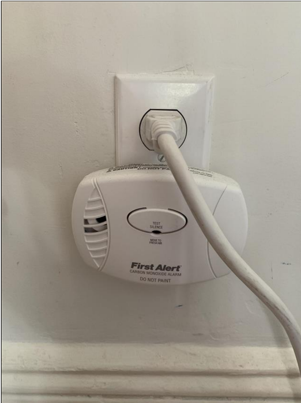
7.8 Item 1(Picture) A few plug-in CO detectors were noted but these may not come with the home.
