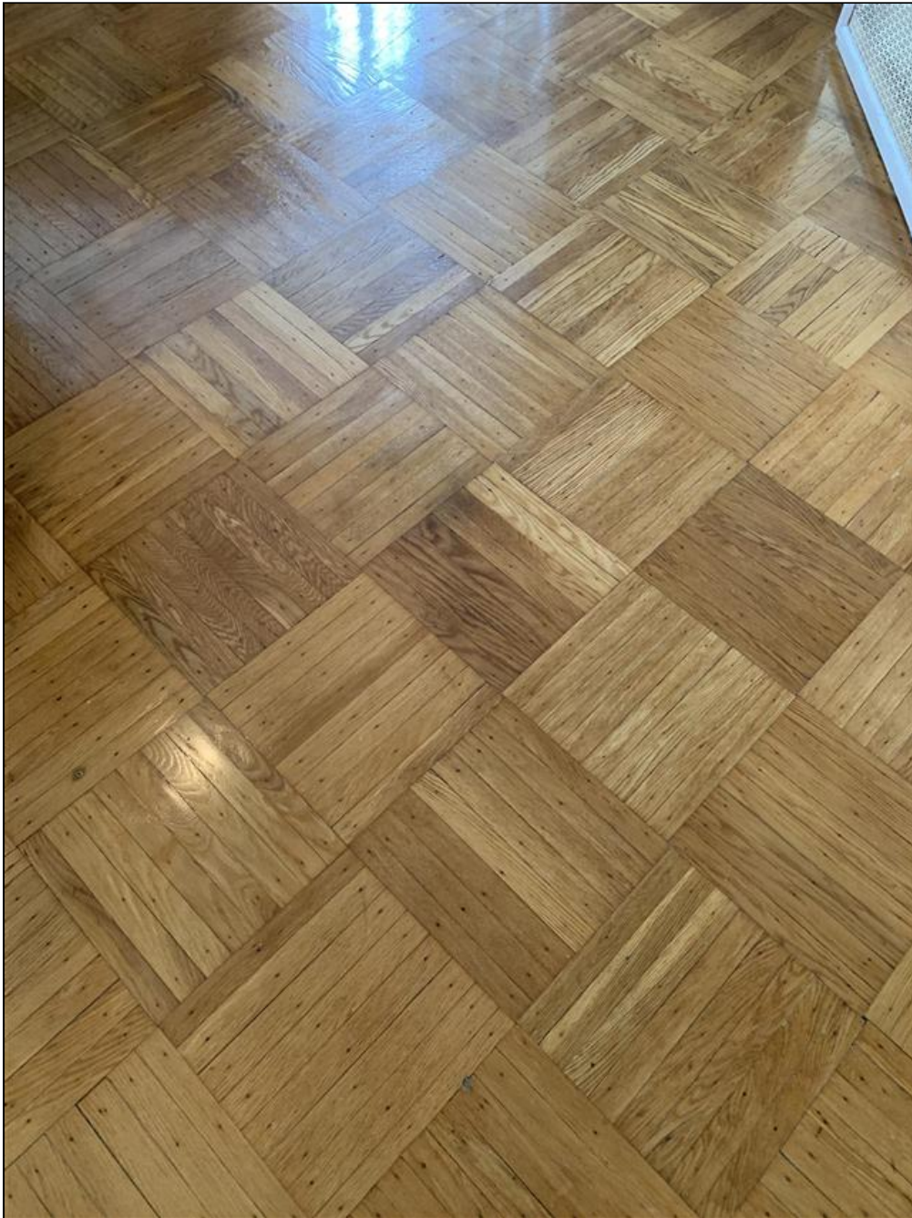
4.2 Item 6(Picture) Second Floor: Example photo of wood flooring.
